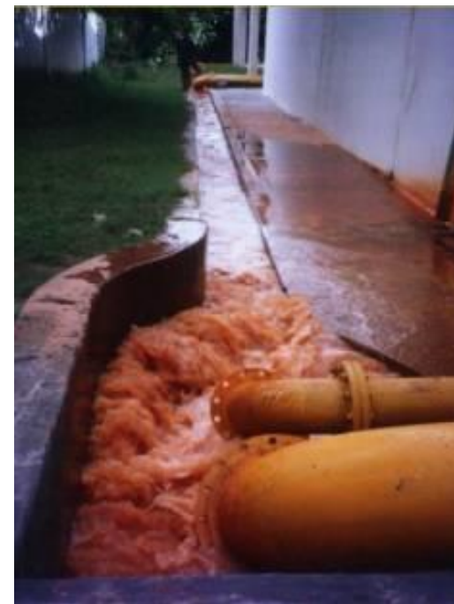
Arsenic sludge from backwashing disposed untreated into Kumar River in Bangladesh
