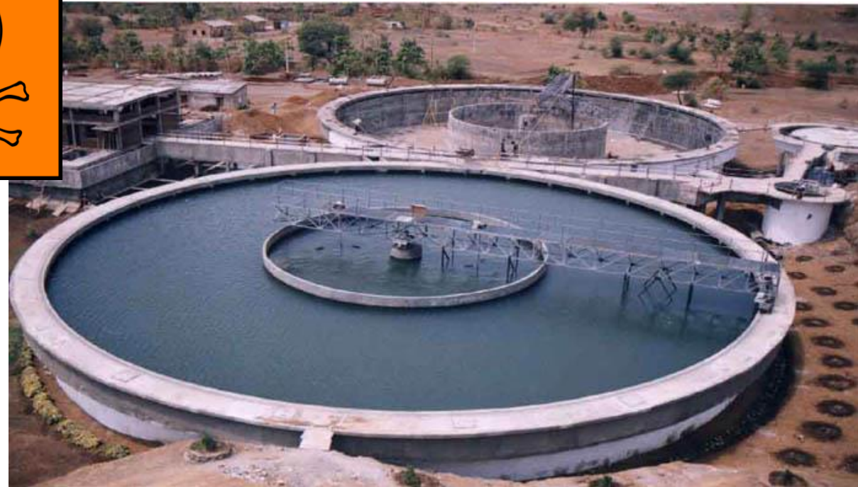
Large flocculation tank in operation
