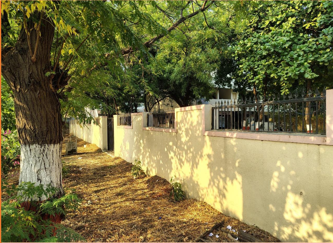
College Compound Wall
