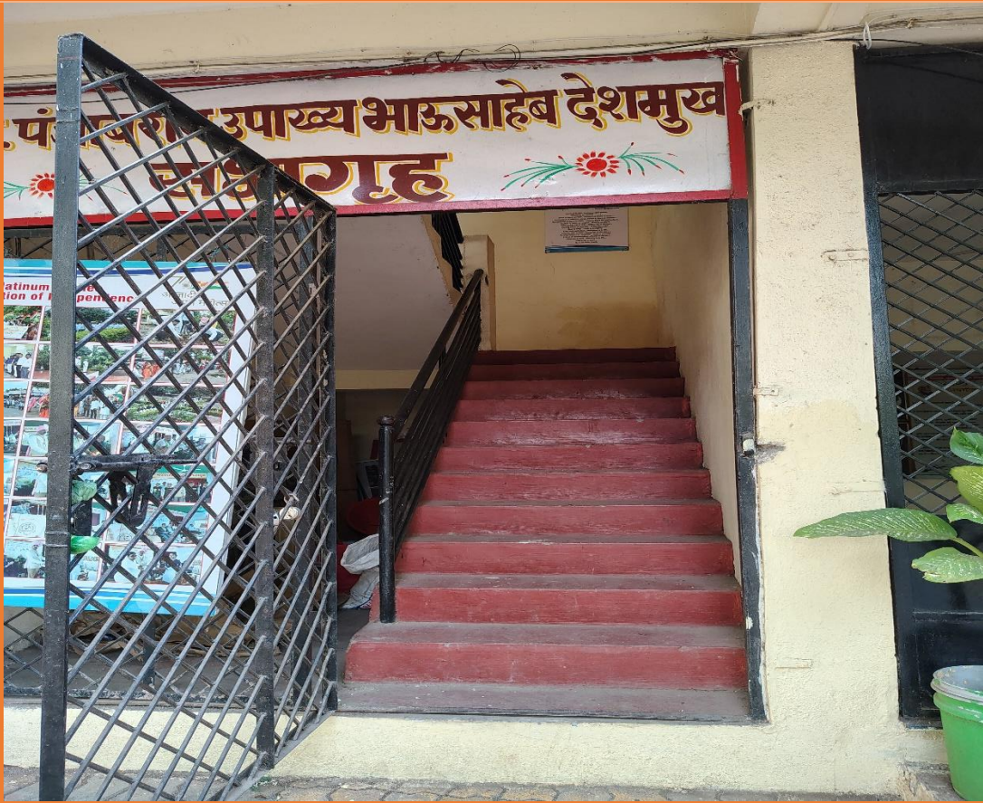
Auditorium Stair Cases
