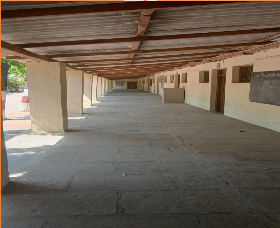
Corridor (Old Building)
